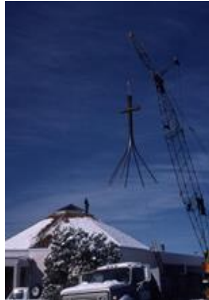
Cross designed by church members being installed.
