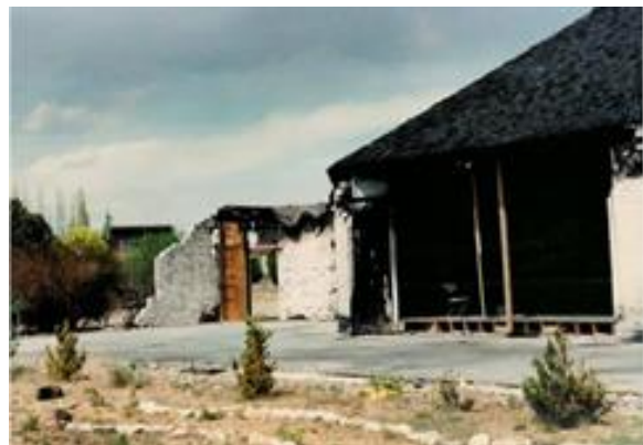
Bryce Avenue Fire Damage in 1992 showing fellowship hall destroyed.
